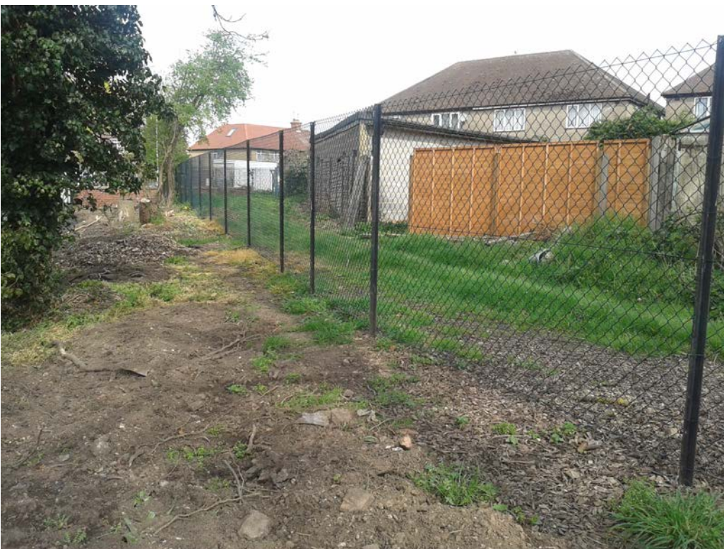
New fencing installed
