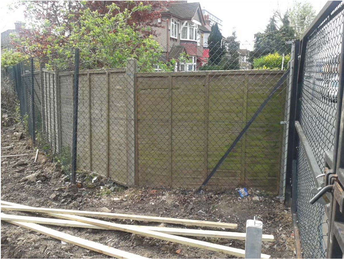
New fencing installed
